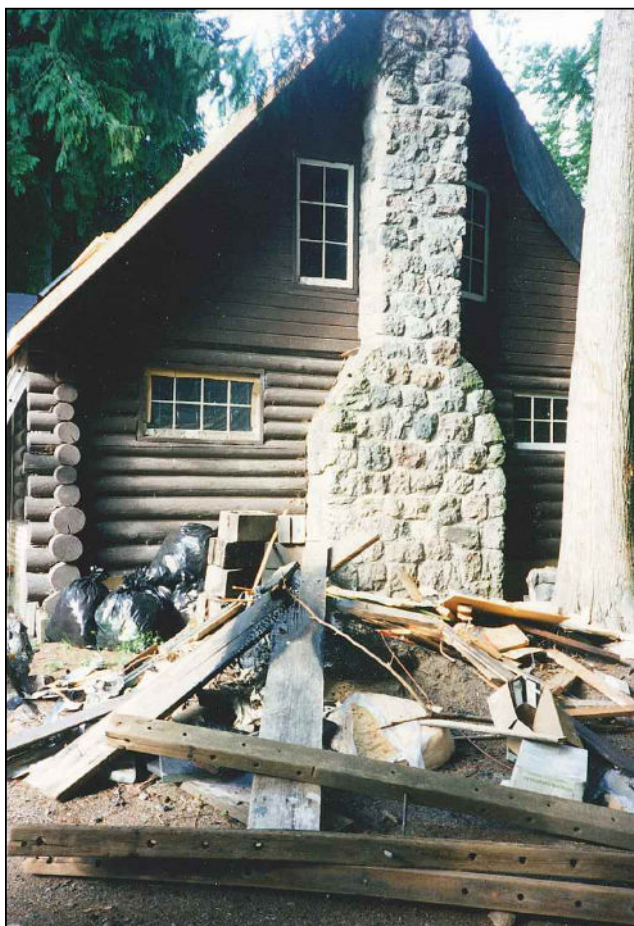
Major clean-up had to take place before the restoration could begin.
